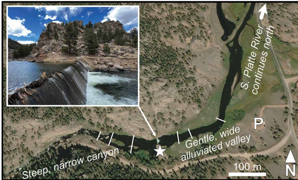
Figure 13. Aerial photograph (© Google Earth, 2020) and field photograph (Lyndsay Saunders, U.S. Forest Service) showing the Lake George Diversion Dam before it was removed. The star indicates the former dam, now the site of the fishing platform from which we will observe the area. Cross-stream lines are the six cross sections where we collected repeat surveys of channel form. Control cross sections are located >2 km upstream (not pictured). The upstream-most cross section is located immediately upstream of, rather than within, the former impoundment. P—parking area.
